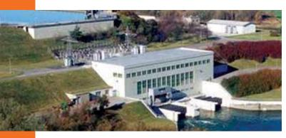
per year. Its renovation is urgent due to the deterioration of unit and turbine equipment. The renovation will also result in increased electricity production and increased safety for people and the environment.
